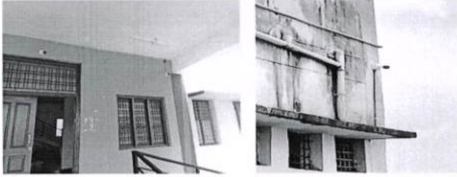
CCTV camera installed in all the Boys hostel (Malaprabha, boys hostel)
