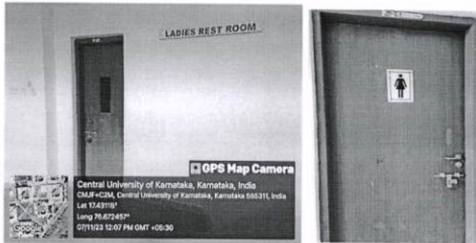
Ladies Rest Room at Each school of the Central University of Karnataka.
